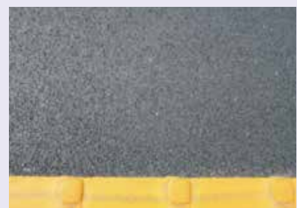
Macadam Mastic Type Finished Surface
