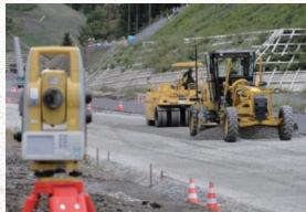
Anti-freezing pavement (Type G Zapeck method)
