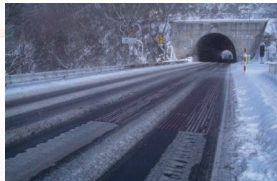
Anti-freezing pavement (Type G Zapeck method)
