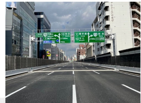
Large-scale pavement repair work (2020-3-Kan)
