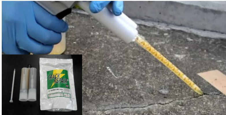
CRACK REPAIR
